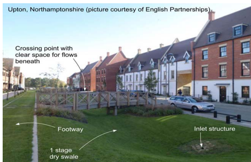
Photo 1: Example of best practice - Dry swale with crossing point at Upton Northamptonshire.
