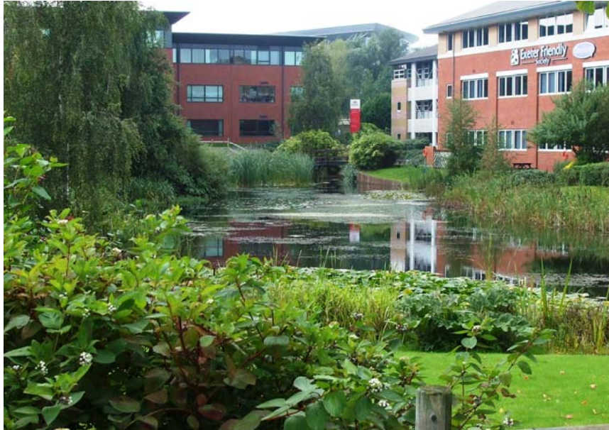
Photo 2: Example of best practice - Wet pond with storage provided above permanent water level at Exeter Business Park, Exeter.
