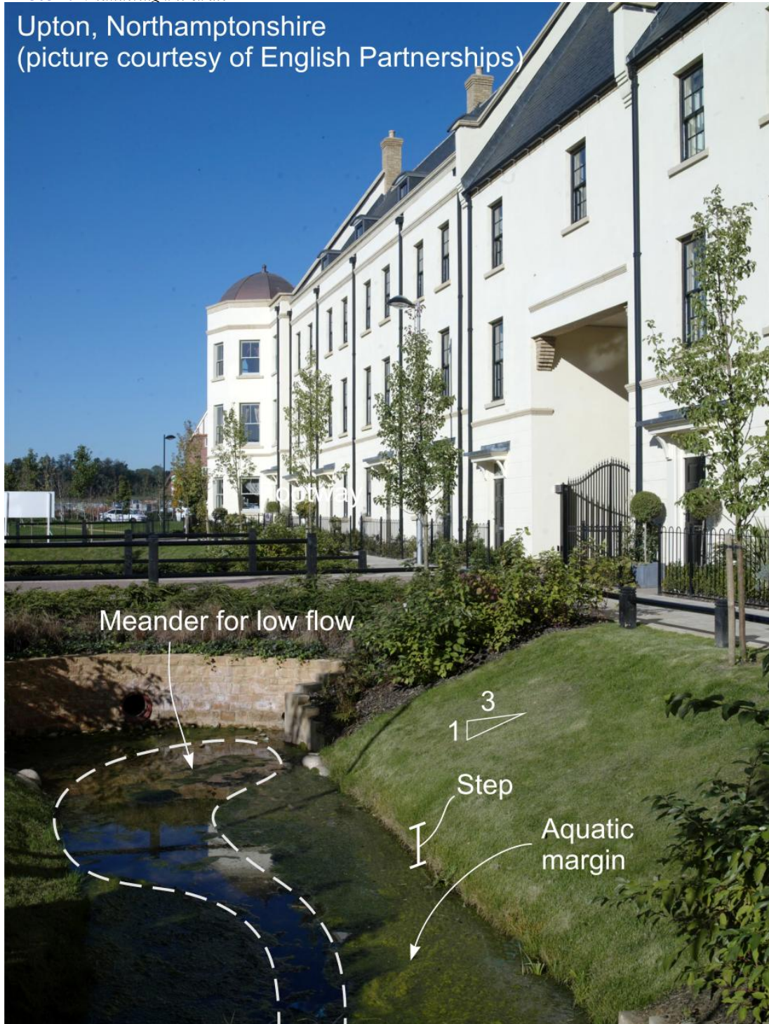
Photo 1: Meandering wet swale
