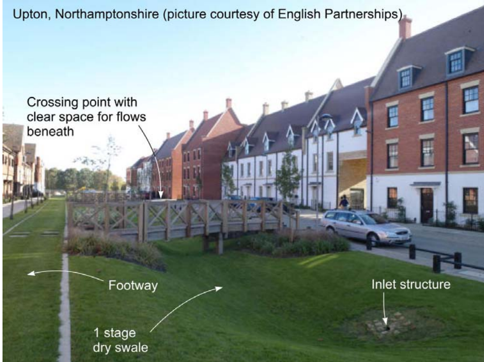
Photo 3: 1 stage dry swale with crossing point
