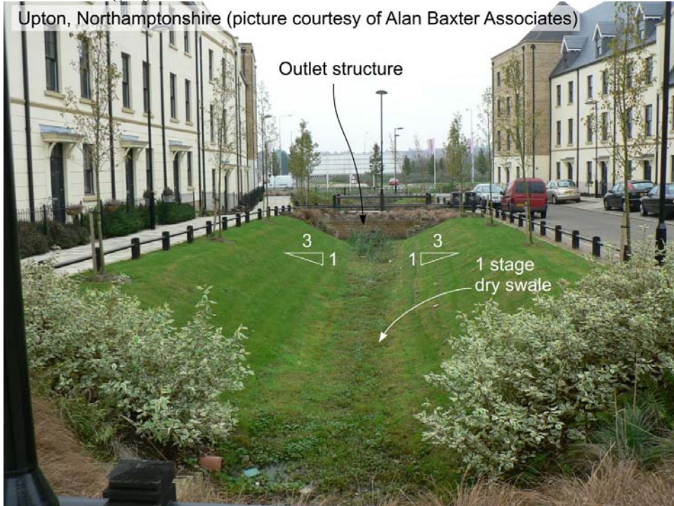
Photo 2: 1 stage dry swale
