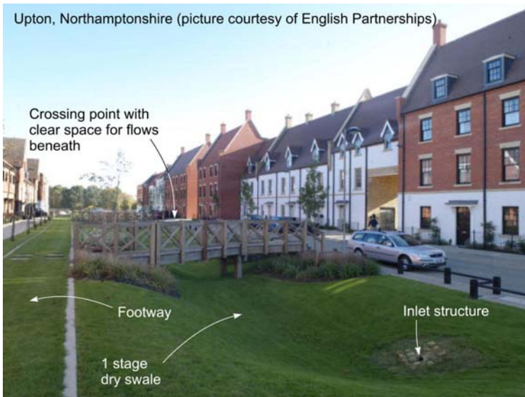
Figure DS 3.0: Dry Swale used For conveyance of storm water and attenuation.
