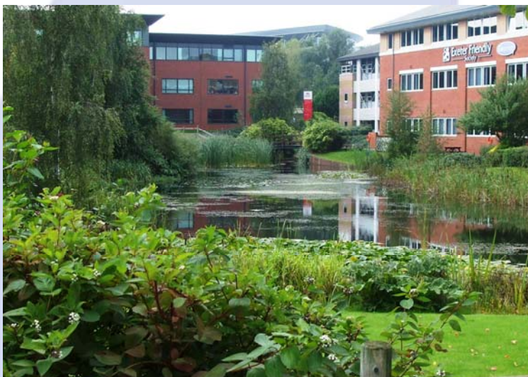
Figure DS 3.1: Exeter Business Park (wet) attenuation pond with storage volume provided above permanent water level.
