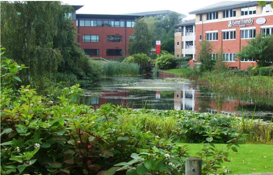
Figure DS 2.1: Exeter Business Park (wet) attenuation pond with storage volume provided above permanent water level.
